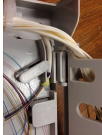
Cable position in the splice tray
